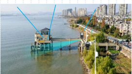
Hydrological Station Management
